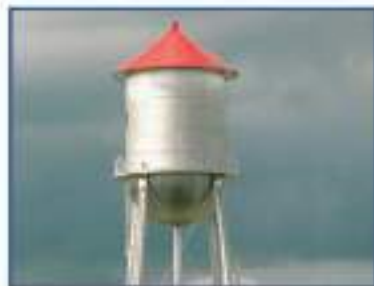
Standpipe (water tower)
