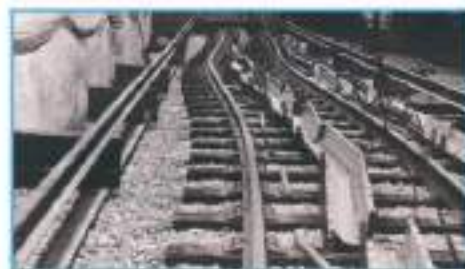
Gaps are placed between railway bars
