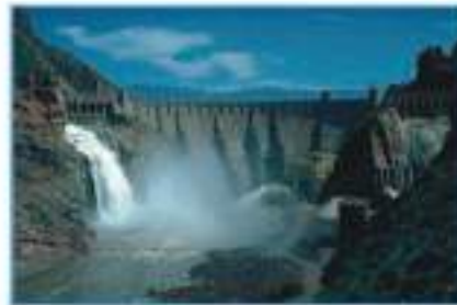
Dams are thicker at the bottom, because water pressure increases as its depth from the surface of the liquid increases.
